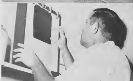
STUDYING A gamma ray film of a pipeline in service in Senior Engineer R. W. Kriek, above. At top, G. J. Crjanovich, senior chemist in TSD-Laboratories, sets up a gamma radiography shot. R. Hodge, EIG engineer, middle photo, is taking an X-ray of a weld.
